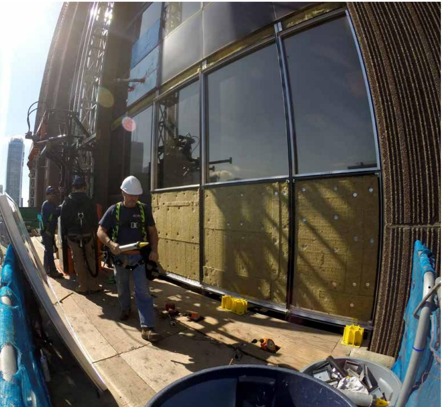
*Overcladding involved leaving existing frames in place and anchoring a new system to the original frames. A new insulated backpan and spandrel panel were included in the new system. The original vision glass was moved to the interior, and the interior of the original frames was overclad.*
